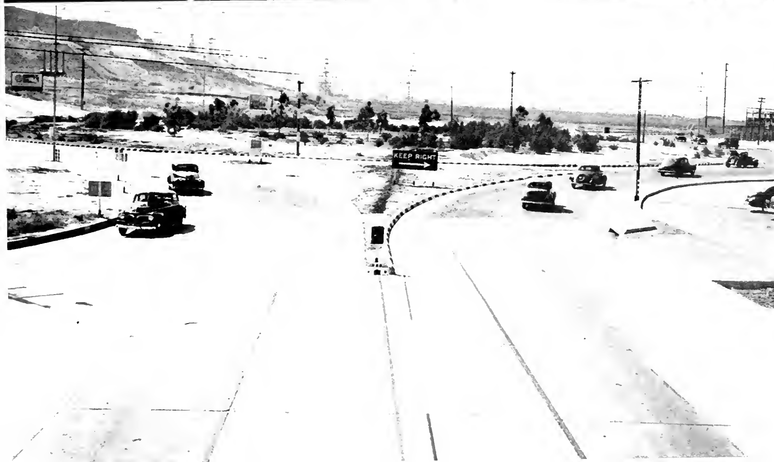
Views of reconstructed traffic circle at intersections of State Street, Lakewood Boulevard and Hathaway Avenue in Long Beach which now consists of a circle within a circle. At top—channelization at State Street entrance. Below—Hathaway Avenue approach
